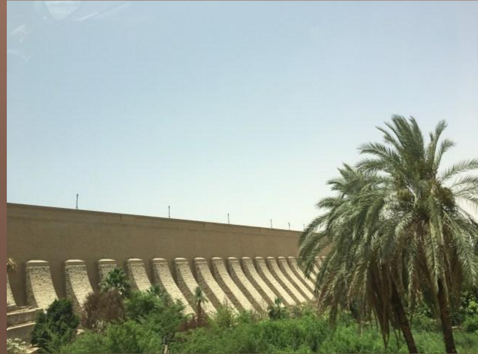
First Aswan Dam Aswan Low Dam Today
